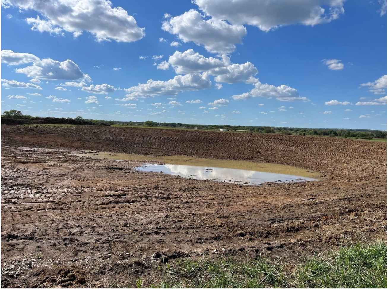
Figure 4. After excavation. (Photo by author.)
