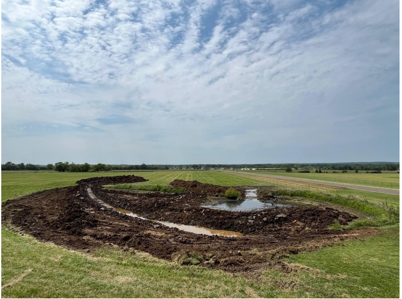
Figure 3. During excavation. (Photo by author.)
